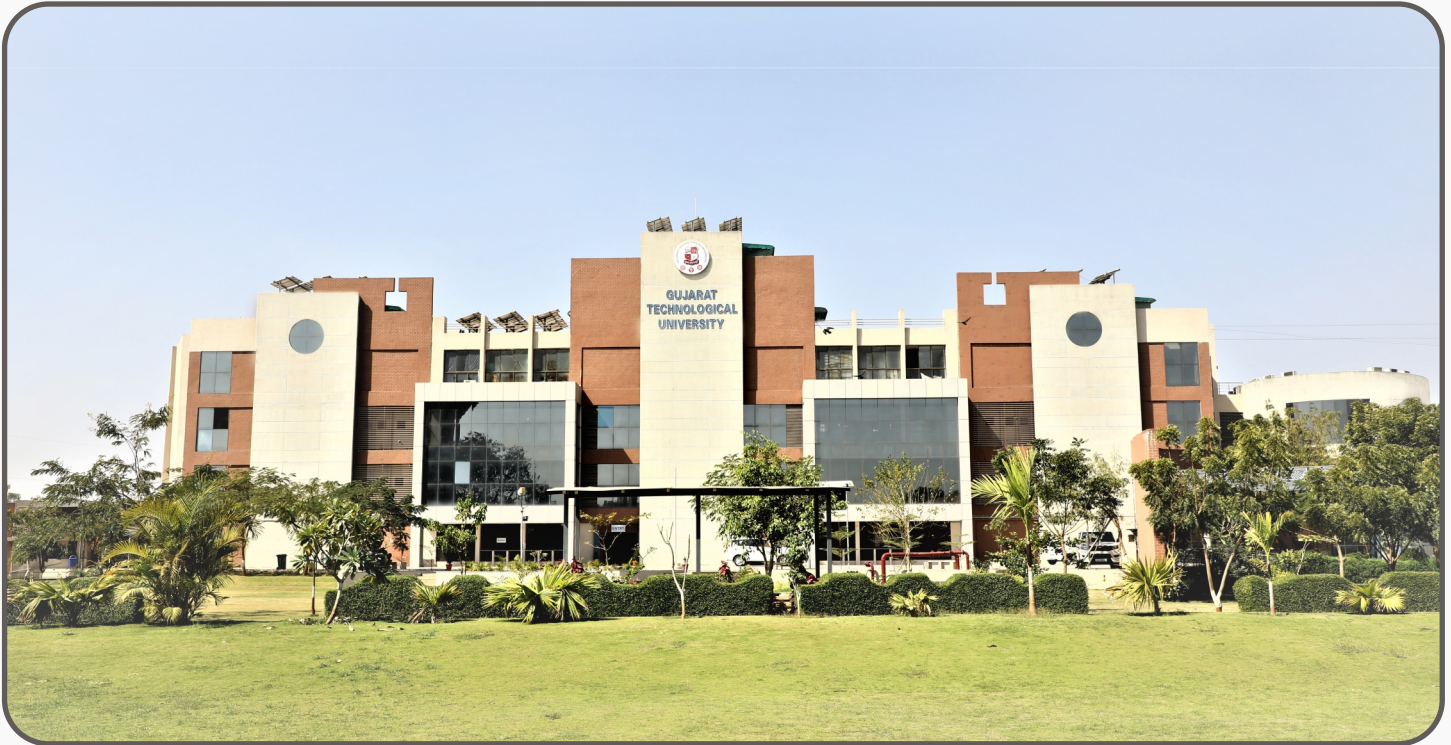
GTU Chandkheda Campus, Ahmedabad
